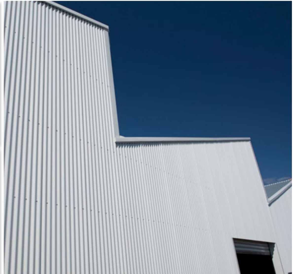
9. Underdale Warehouse COLORBOND® Steel Surfmist®
